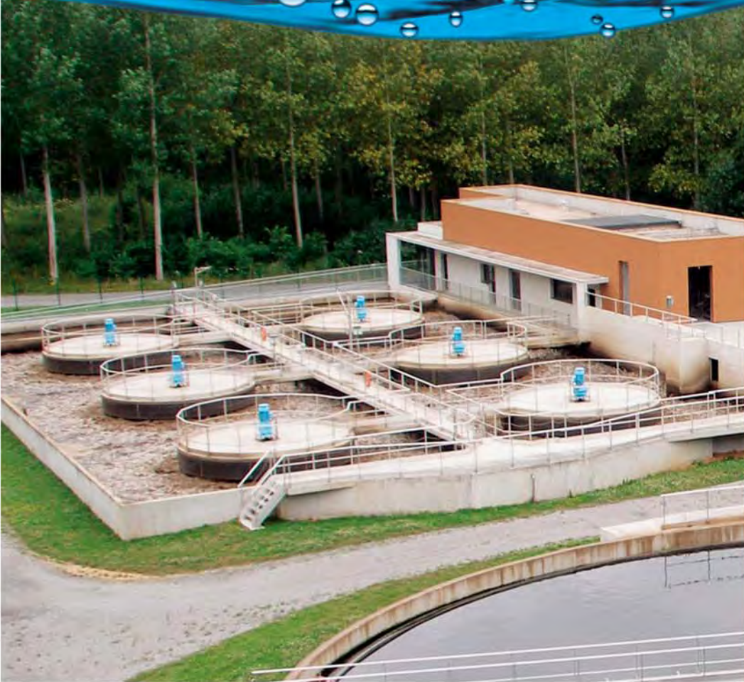
Station d'épuration urbaine Municipal treatment plant
